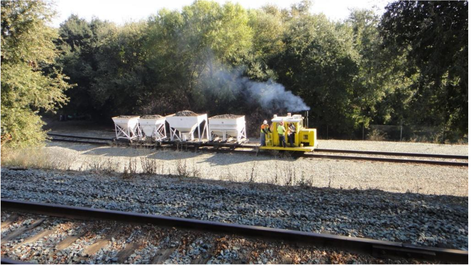
Frank pilots the ballast train, filled with 12 tons of rock, up the Setzer Grade. Luckily, Mike F (on the back deck) took a look at the coupler...
