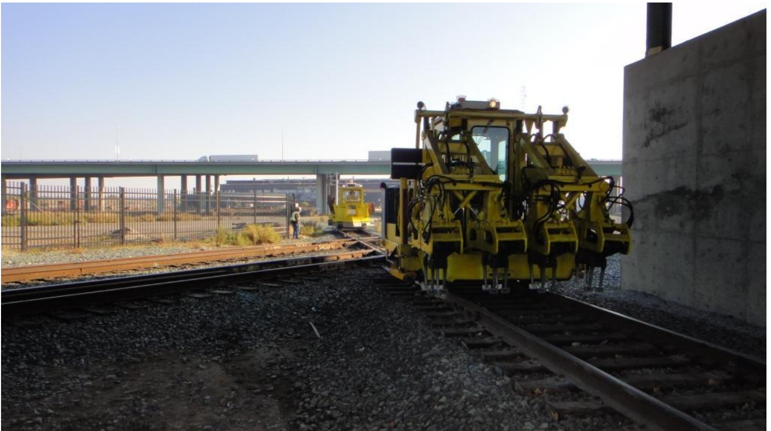
Conductor Frank conducts the tamper and ballast regulator across the UP Main on Saturday morning
