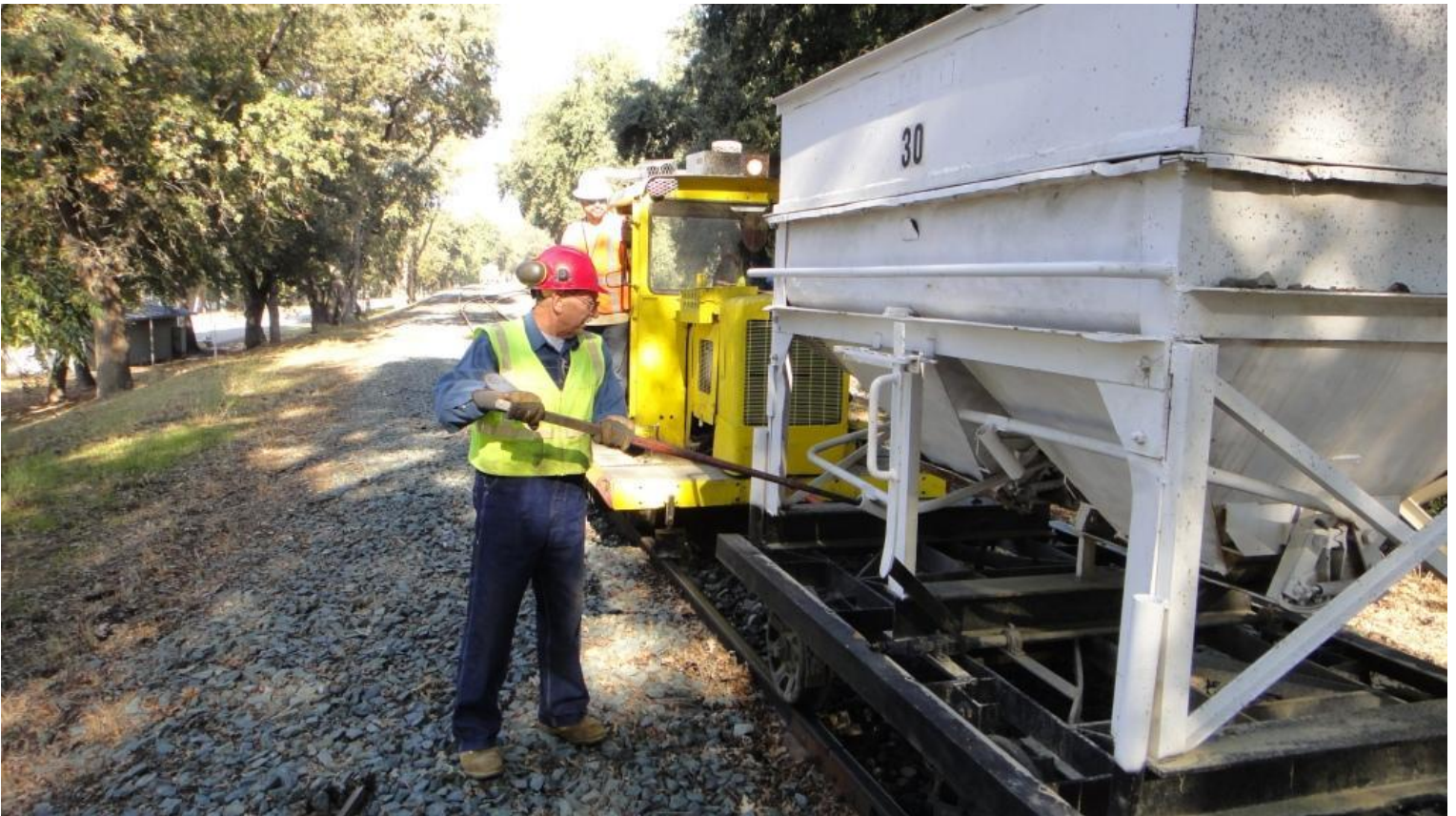
Clem disgorging rock from the busted ballast car after the tug ran-around it to hook-up to the coupler on the other side which was still OK
