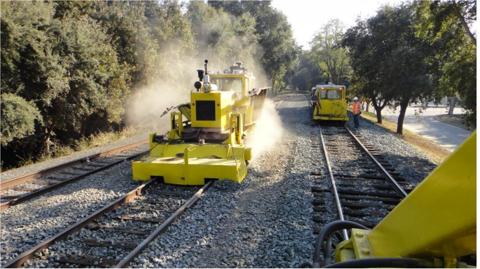
Chris brooms the track with the ballast regulator
