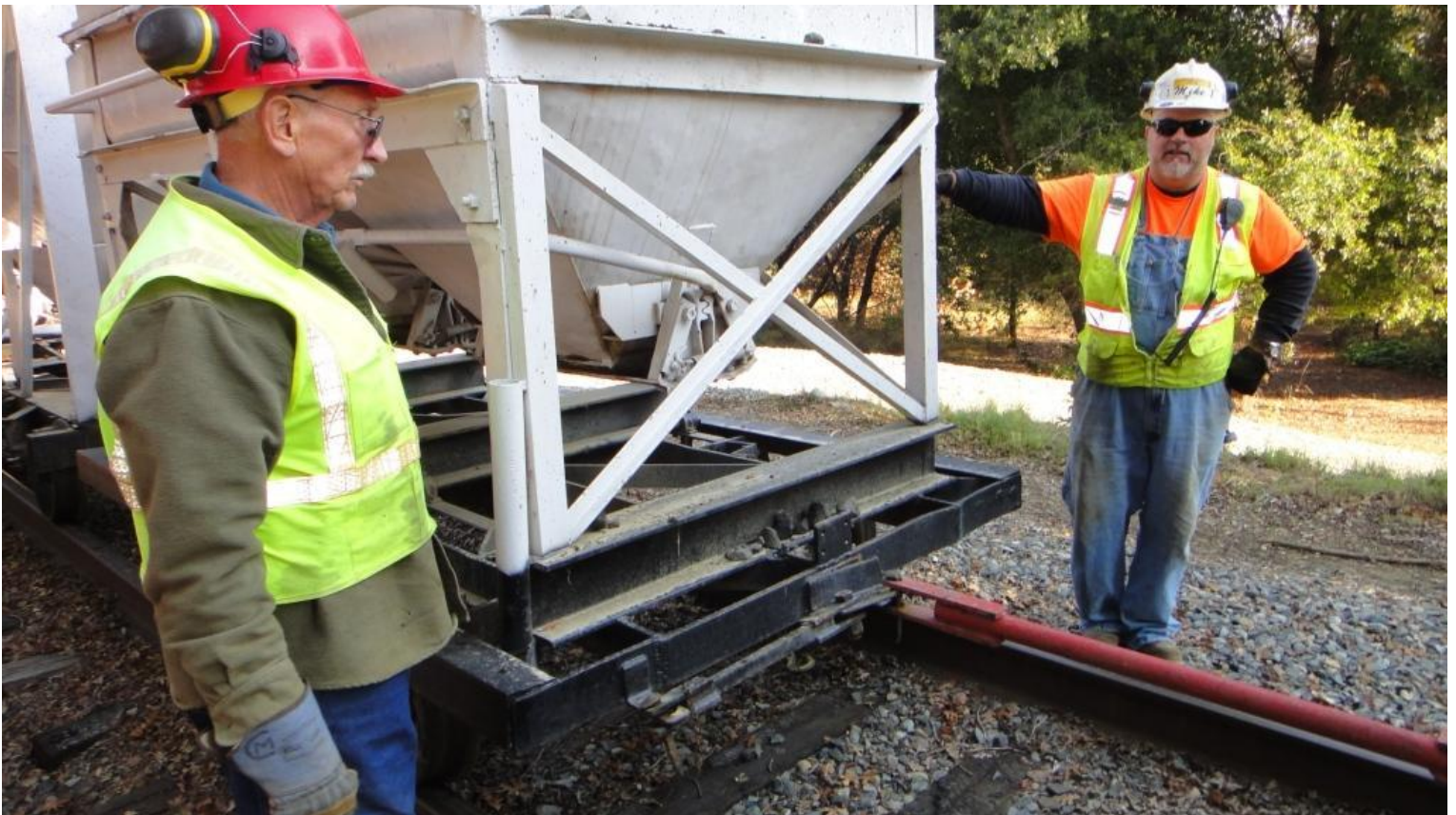
Yeah, this could be a bit of an issue. Clem and Mike F. survey the broken weld on the center-dump ballast car's draw-bar coupler
