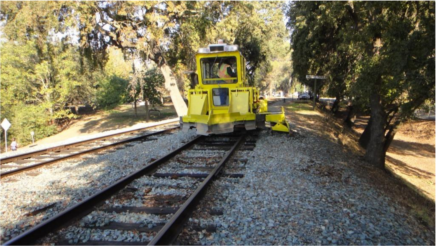
On the Miller Park siding, Chris deploys the short-side wing on the ballast regulator
