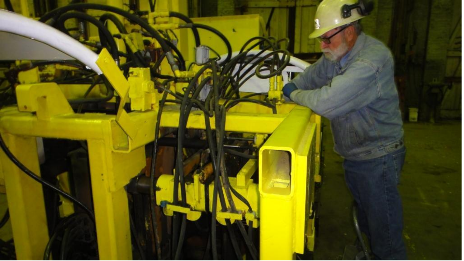
Alan works to install the newly repaired hydraulic cylinder on the Super B spiker
