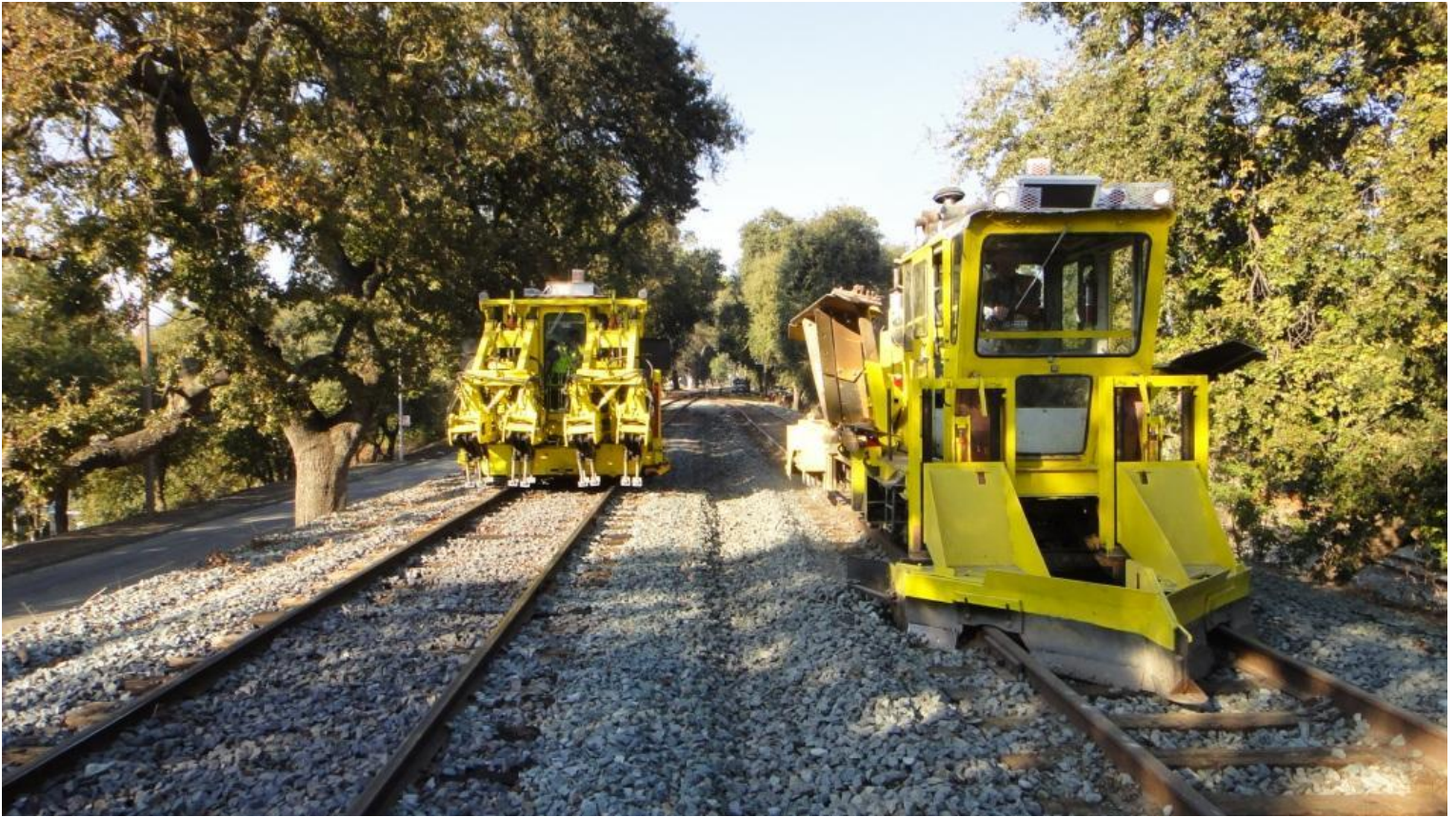
Chris makes a final pass plowing the Miller Park Siding
