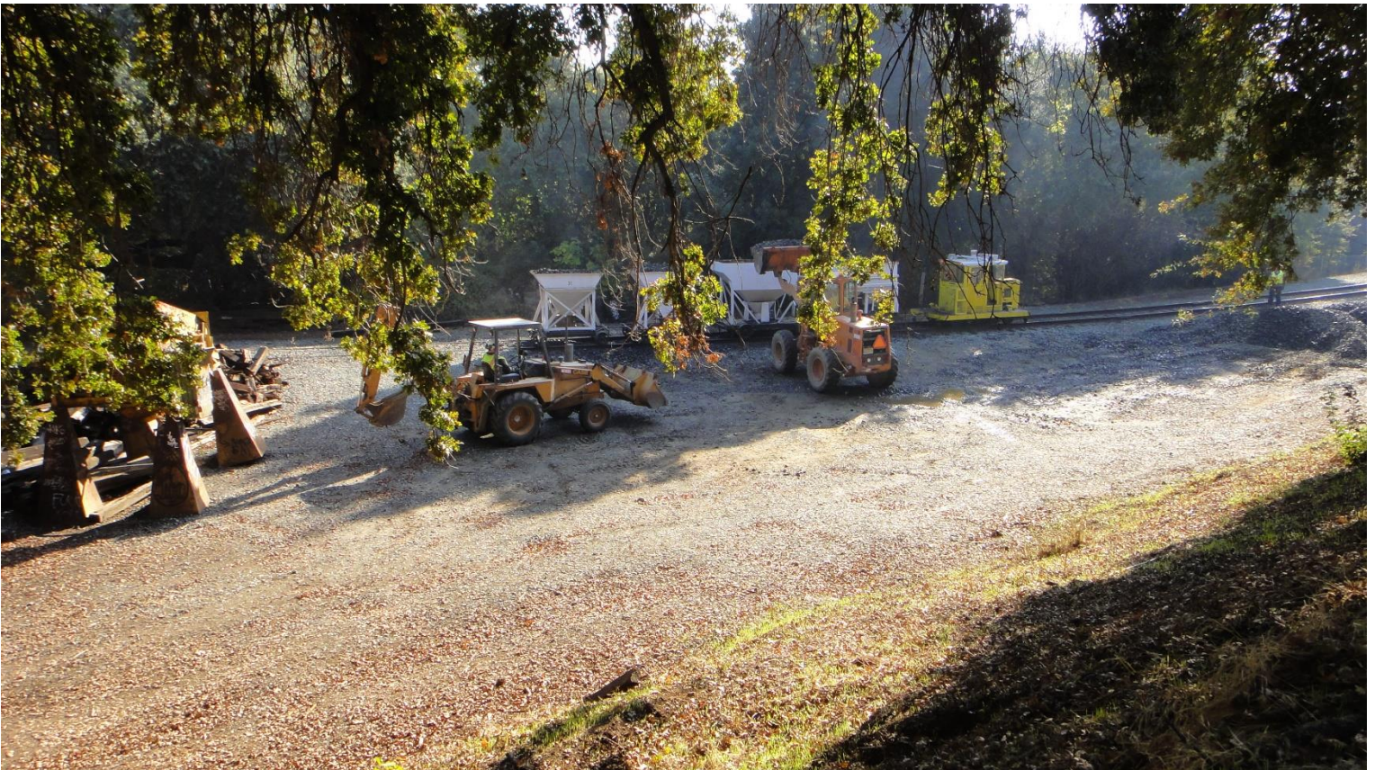
Down in the Setzer Yard, Harry in the back-hoe and Mike F. in the front-end loader fill the ballast cars with rock
